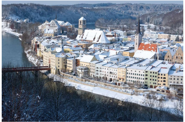
© Stadt Wasserburg am Inn
